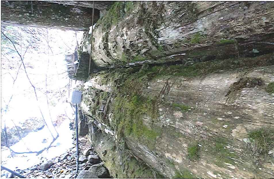
CK2315 Left Abutment
